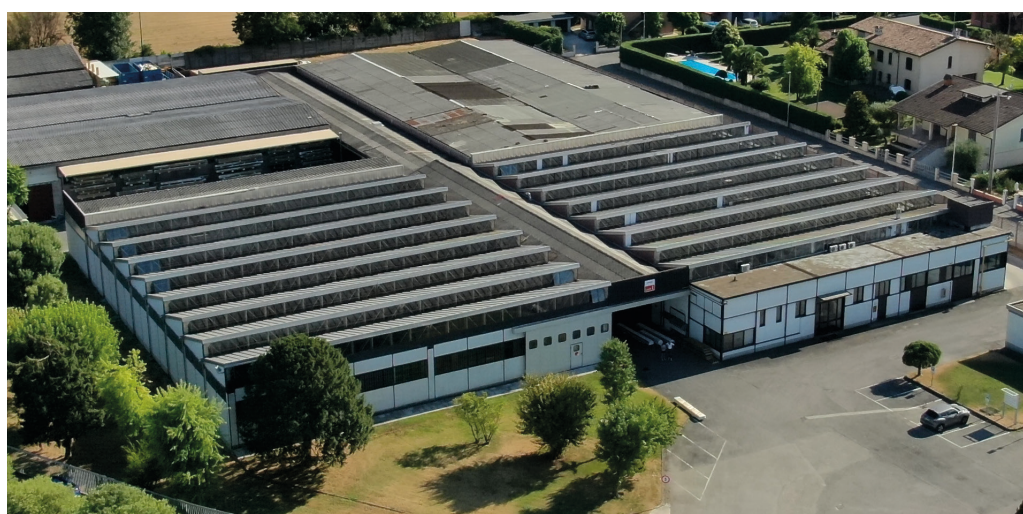
REMEDELLO (BS) PRODUCTION PLANT
